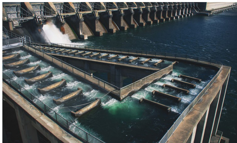
The fish ladder at John Day Lock and Dam that allows adult fish to migrate upstream of the dam.
